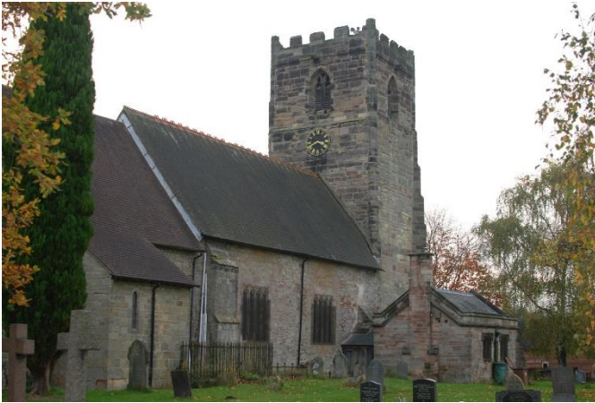
Figure 4.3: Church of St. Laurence, Walton-on-Trent, looking southwest
