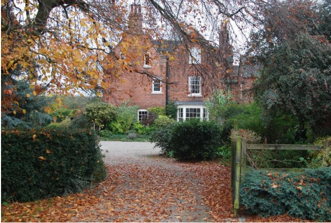
Figure 4.1: Park Farm, looking southeast
