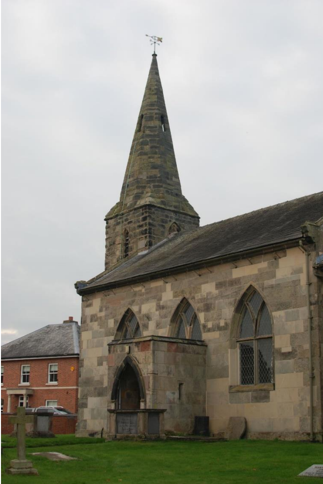
Figure 4.8: Church of St. Mary, Rosliston, looking northwest
